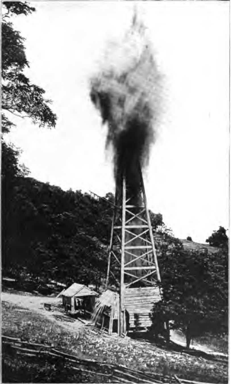
PLATE VIII.—Effect of Shot on a Fifty-foot sand Oil Well in Shinnston pool—Hartley Heirs No. 1 well.
